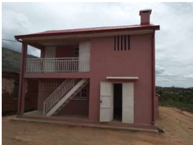
The electricity kiosk and the responsible
